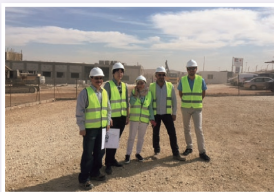
Monitoring the progress of a construction of moderation center for counter-extremism in Jordan
